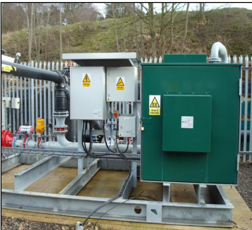
Control panels are pre-wired & tested to speed installation and commissioning & Acoustic housing to minimise noise
