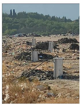
They maintain the verticality of the pipework, the landfill gas enters the wellheads and is been extracted much more efficiently while we can easily plug in a horizontal pipework and lead the landfill gas to the combustion at any time. Optional, they may allow the installation of leachate pumping system simultaneously with the extraction of landfill gas, they may be fitted with flow valves, sampling and monitoring points for leachate level, pressure measurement and landfill gas composition.
