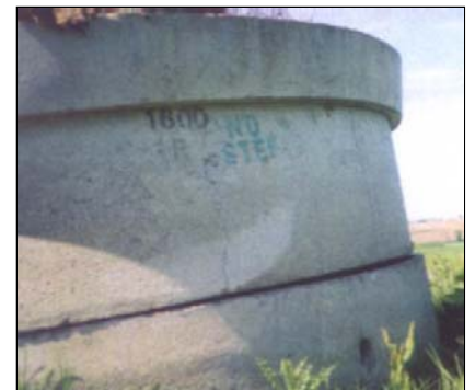
CONCRETE RINGS TILTING
