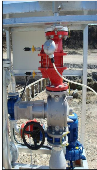
Flame Arrester electric operated safety shut-off valve
