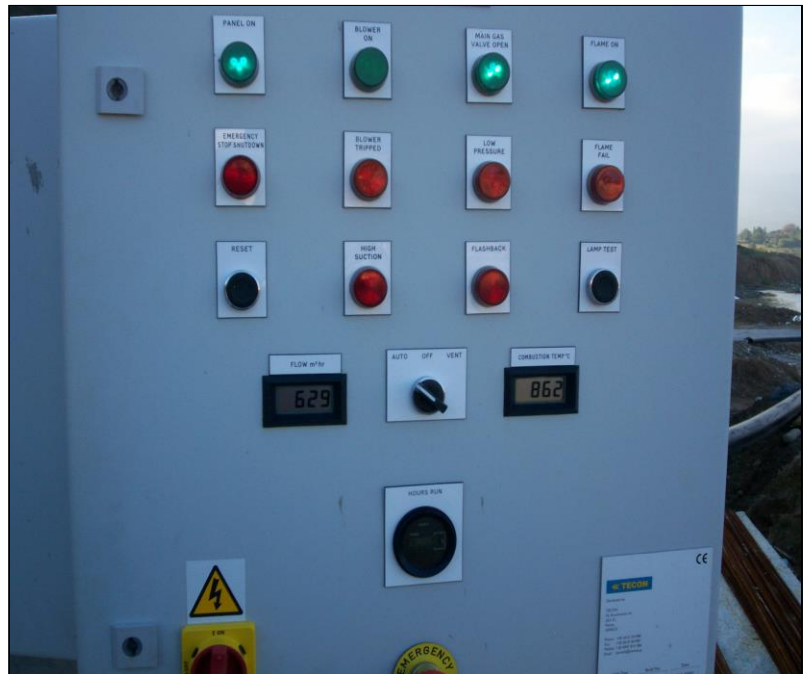
Control Panel c/w Flow & Temp digital display
